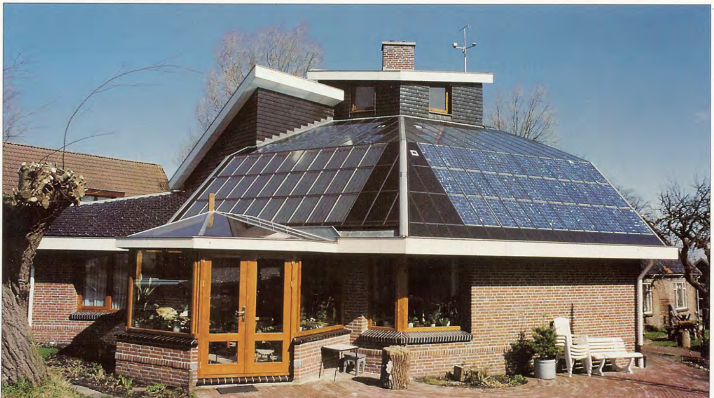
The zero-energy house in Woubrugge.
